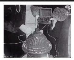
Here are some photos of the world's first cell phone in use. This happened in Britain in 1922. Note the phone had to be grounded to the fire hydrant and the antenna was fastened to the umbrella.
